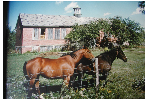
Falls Into Disrepair
